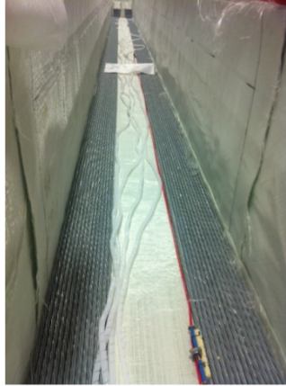
Figure 8 - Internal VWG Placement at Tension Level
